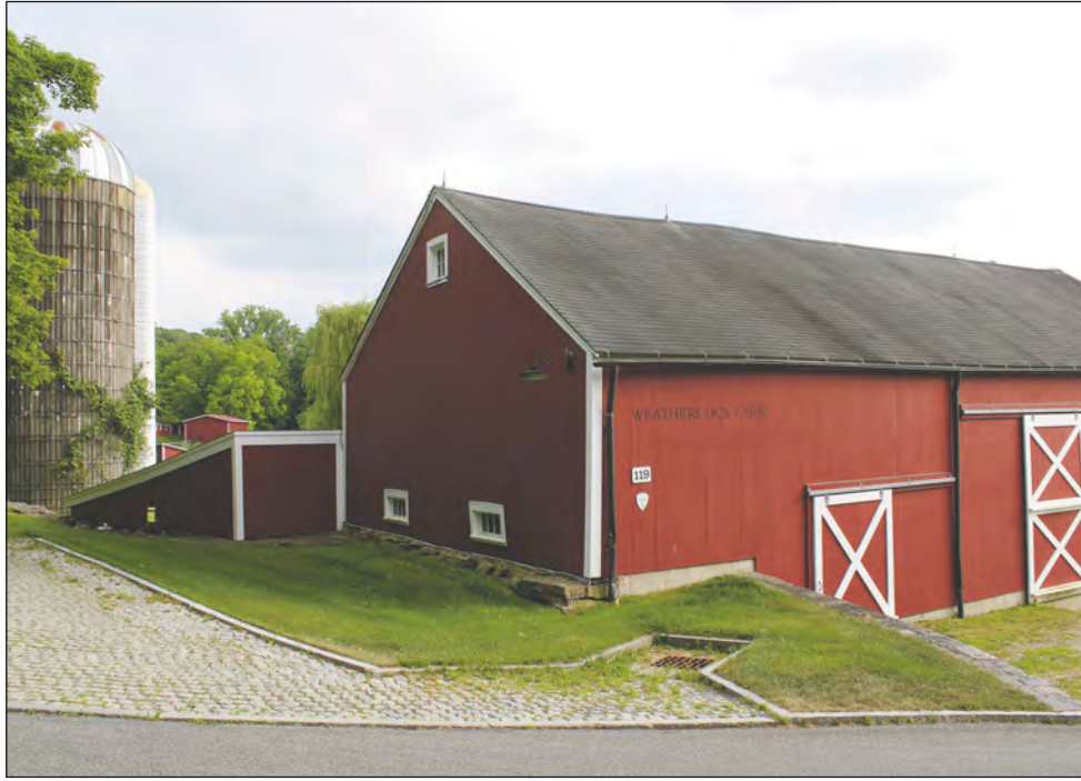
A barn and silo on Calkinstown Road in Sharon.
