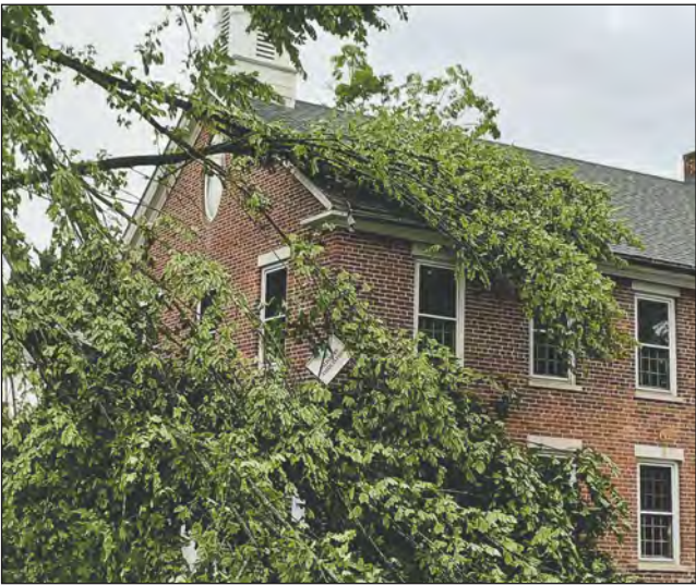
Left: A tree falls on the historic Academy Building, which houses the Salisbury Association. Right: Resident Ben Blackwell directs traffic in Salisbury as motorists navigate road closures.
