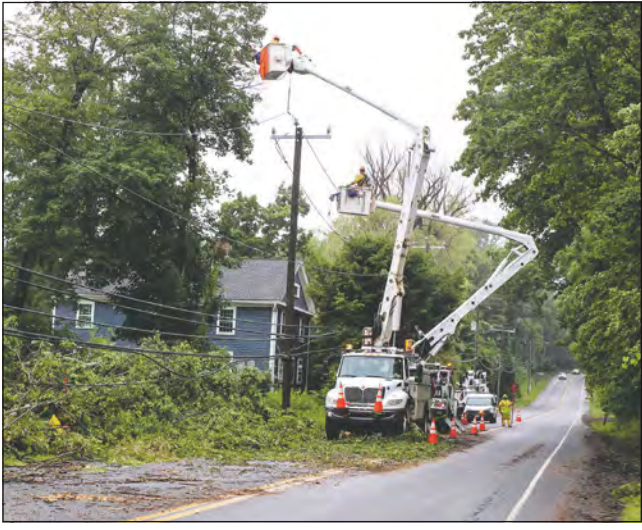
A crew working on a downed tree and utility pole in the westbound lane of Route 44 east of Cobble Road on Tuesday, July 7.
