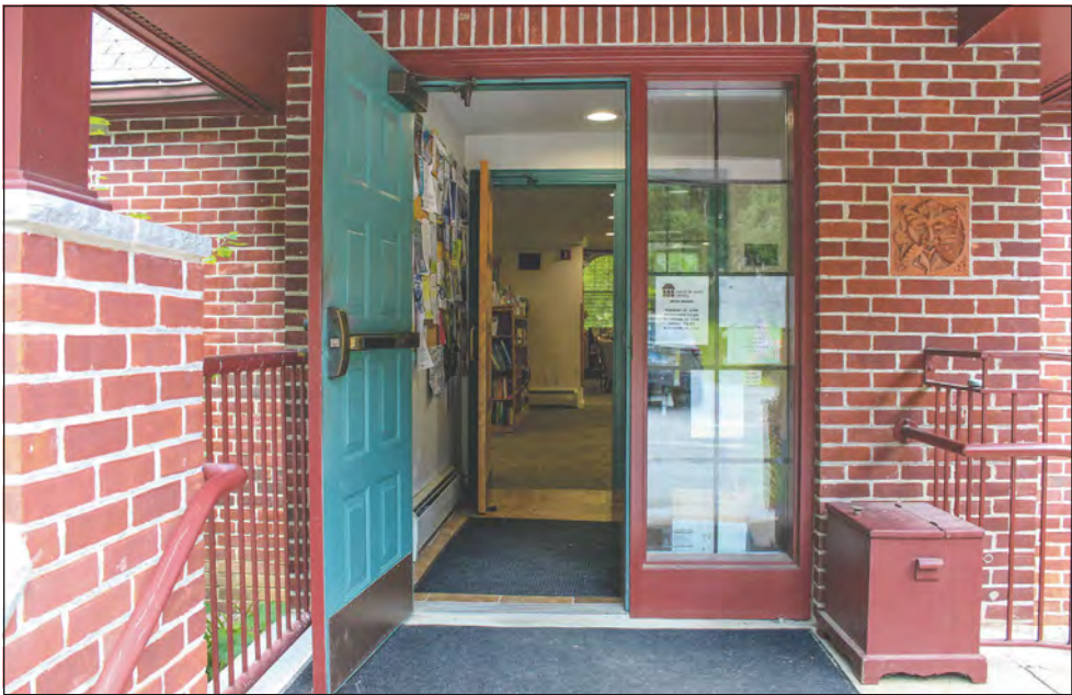
The Hunt Library could receive automatic doors thanks to a $10,000 grant from the American Library Association.
