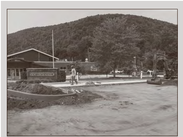
PHOTO BY RUTH EPSTEIN An expansive repaving and sidewalk replacement project at Kent Center School is expected to be completed by the new school year.
