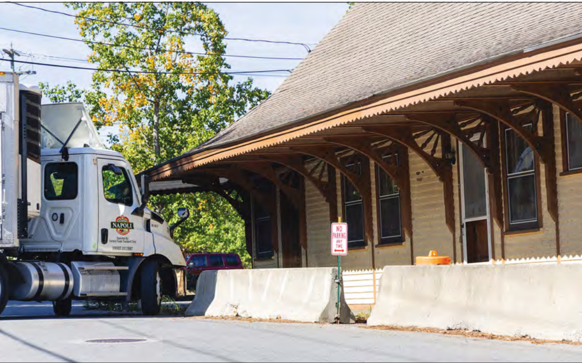
A delivery truck strikes the overhanging roof of Lakeville's historic railroad station on Ethan Allen Street on Monday, Sept. 21. The collision came five days after voters approved spending up to $650,000 to move the building back 19 feet from the roadway.
