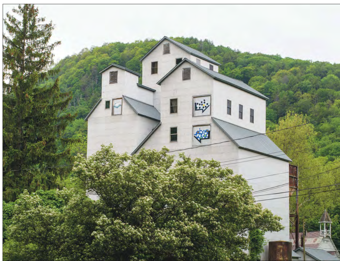
PHOTO COURTESY WASSAIC PROJECT
