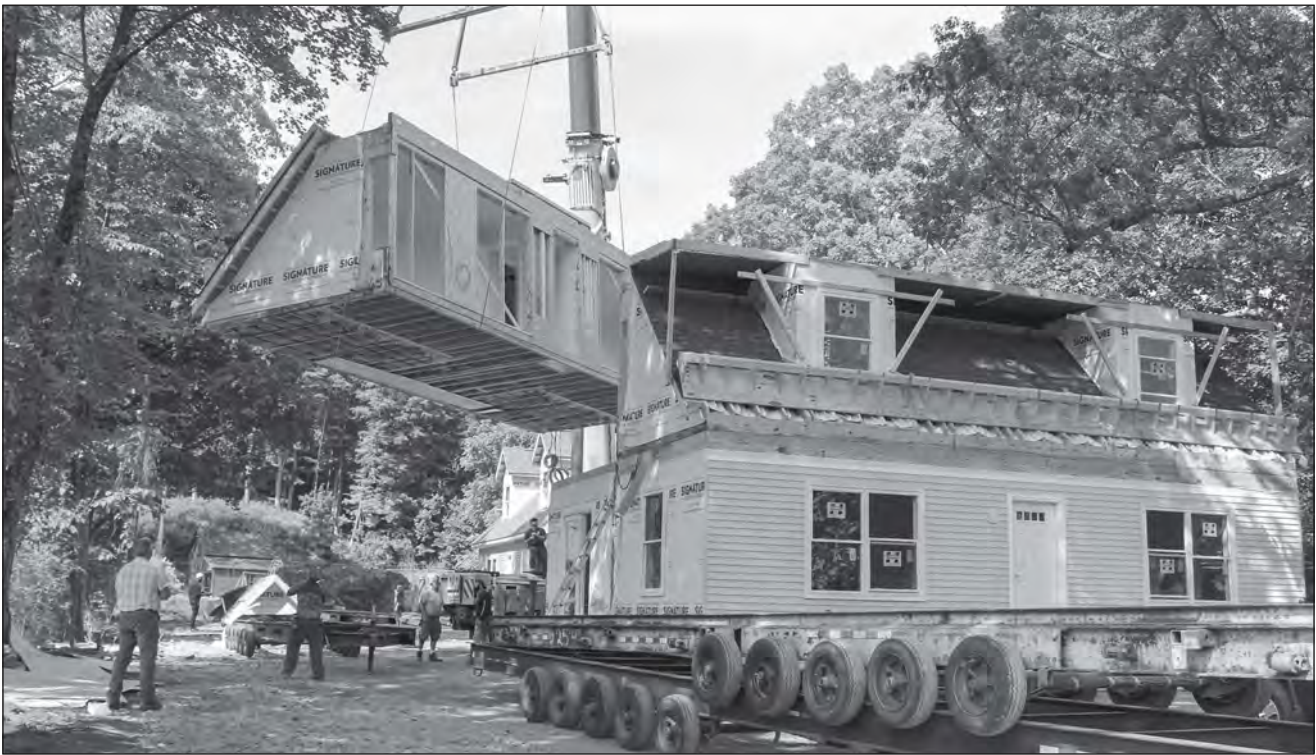
A crane crew carefully installs the second story of a future affordable home on Undermountain Road.
