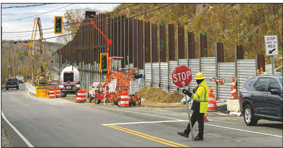
PHOTO BY JENNIFER ALMQUIST Traffic on Route 44 in Norfolk remains reduced to one lane as construction continues on the large retaining wall. “As a team, we are saddened to see First Selectman Riiska leave his position but are looking forward to working with the incoming First Selectman Henry Tirrell to bring this project to success.” To report a problem or raise a concern, call 860-594-2560 or email: DOT.CustomerCare@ct.gov
