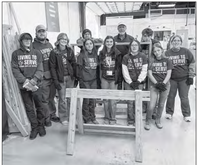
Housatonic Valley FFA built wheelchair ramps for homes during the FFA convention.
